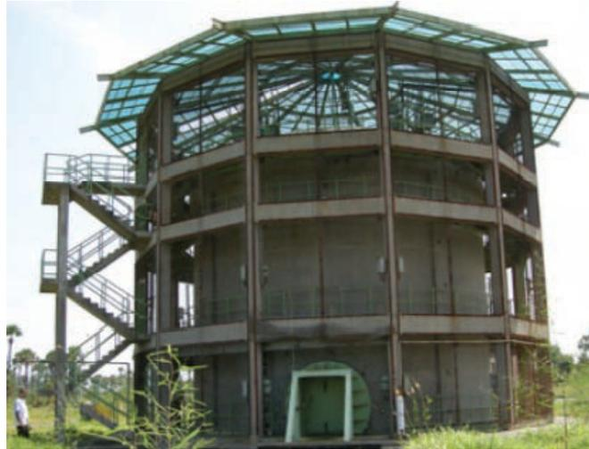
BARCOM, a 1:4 size containment test model at Tarapur is built to generate database of containment performance evaluation studies and
